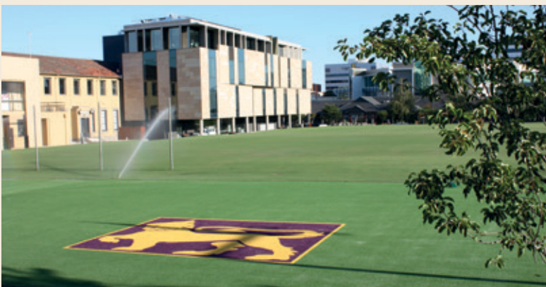
WATER CAPTURE AND STORAGE AT THE ST KILDA ROAD CAMPUS ENABLES THE IRRIGATION OF SPORTS FIELDS, TURFED WITH DROUGHT TOLERANT GRASSES
