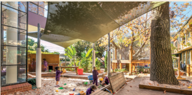
WITH A 100KW PHOTOVOLTAIC SYSTEM, ELECTRICITY USAGE AT THE ELSTERNWICK CAMPUS IS OFFSET BY ELECTRICITY GENERATED INTO THE SYSTEM, WHILE PASSIVE SUSTAINABLE DESIGN FEATURES REDUCE ENERGY USAGE
