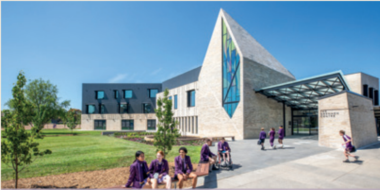
THE DRENNEN CENTRE AT THE GLEN WAVERLEY CAMPUS GAINED A GREEN STAR CERTIFICATION RATING OF 4 – REPRESENTING BEST PRACTICE – FROM THE GREEN BUILDING COUNCIL OF AUSTRALIA IN 2019
